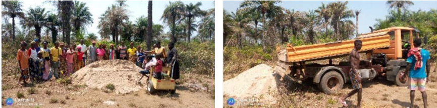
Figure 10: The community prepares the land for building
